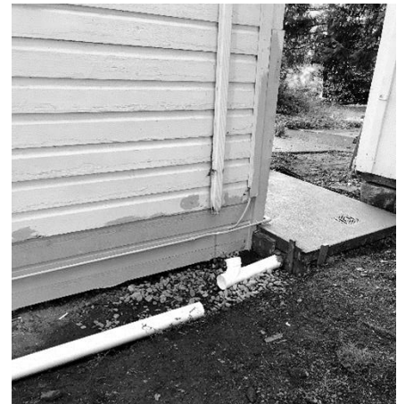
New drains and foundation repair
